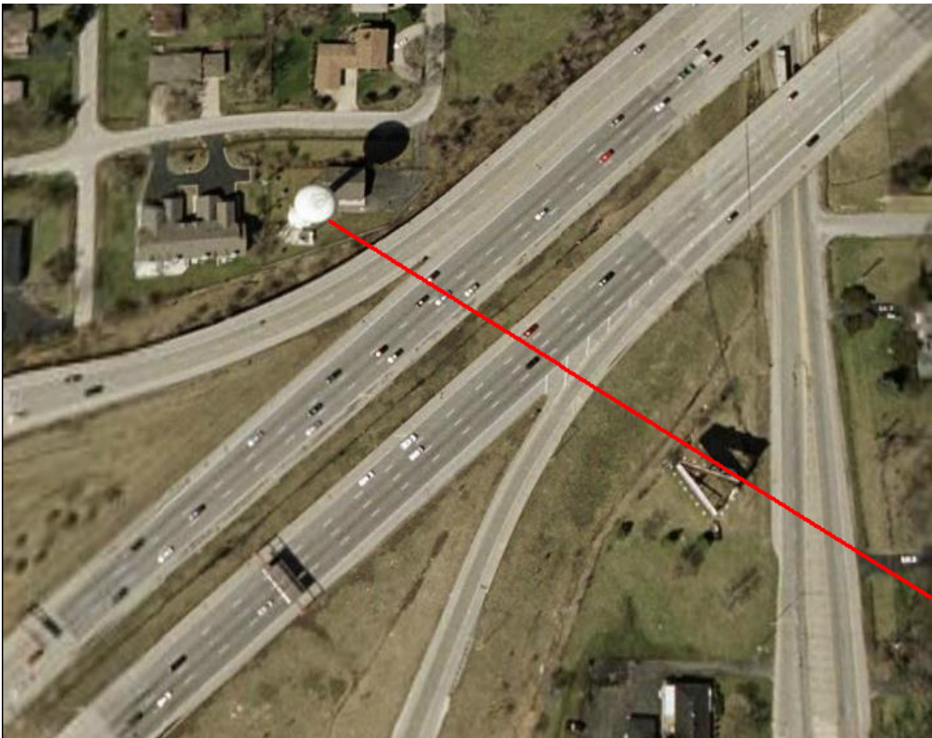
Figure 4 – Microwave link, aerial view
